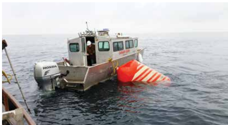
Figure 5. 60-inch brush pig being readied for tow back to shore
